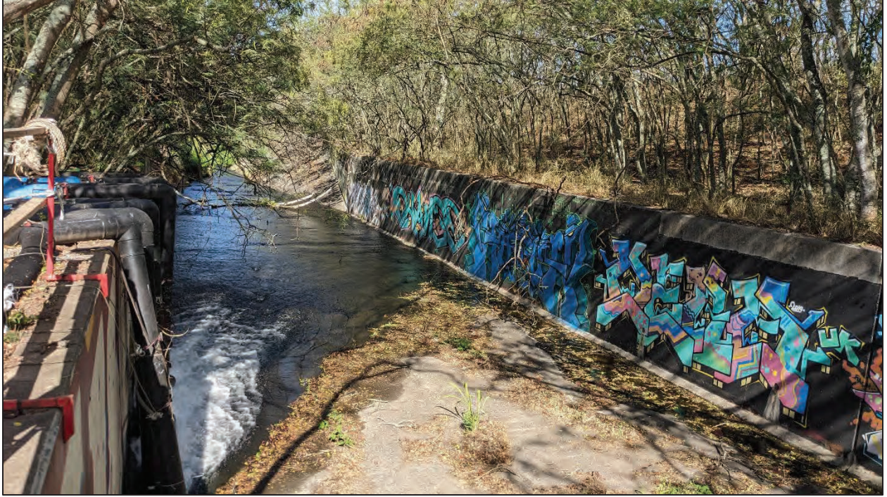
Figure 6. South Halawa Stream in the Project Area Showing Discharge from the Emergency Water Treatment Facility
